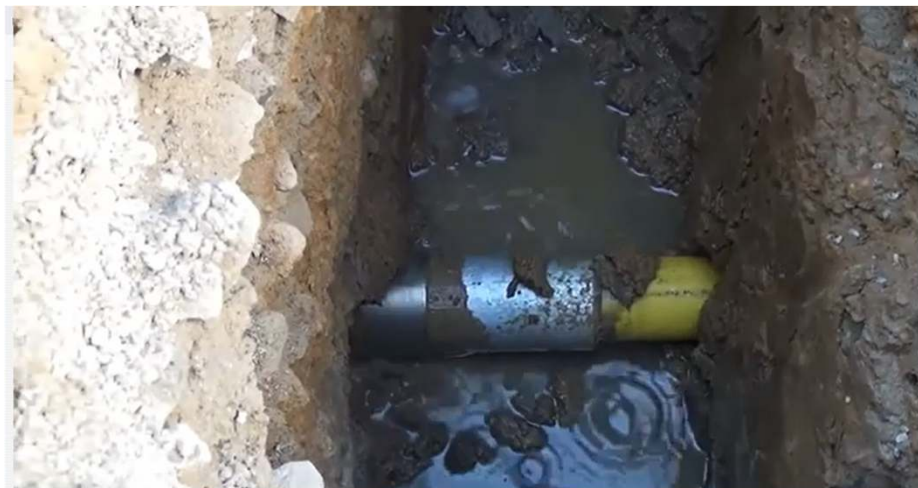
Arrival of the bore head in the control pit
