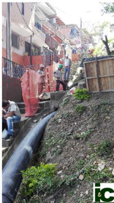
Colector alcantarillado 8" → Pipe Bursting 10"
