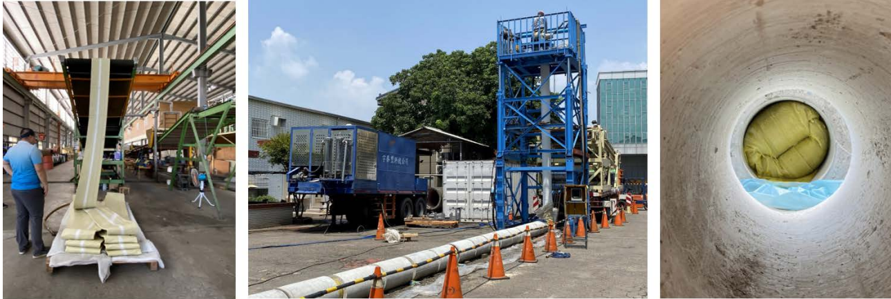
RCPs layout and liner curing.
