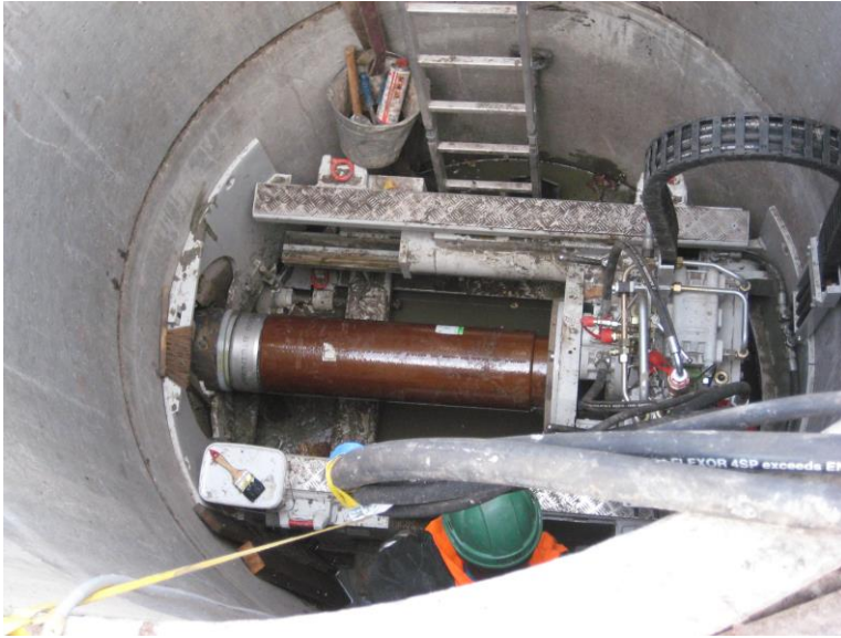
BM400 in 2 m round launch shaft 1 m long product pipes
