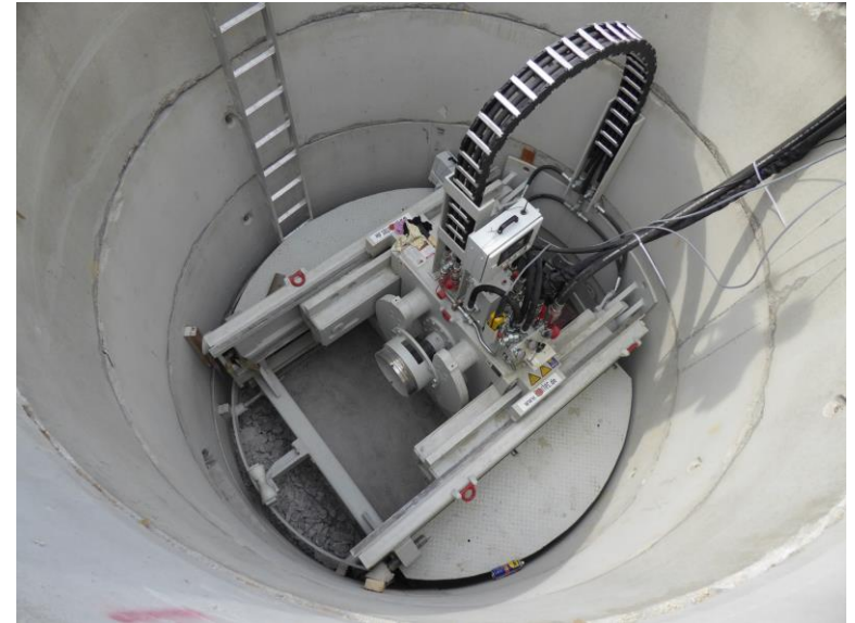
BM500 in 3,2 m round launch shaft 2 m long product pipes
