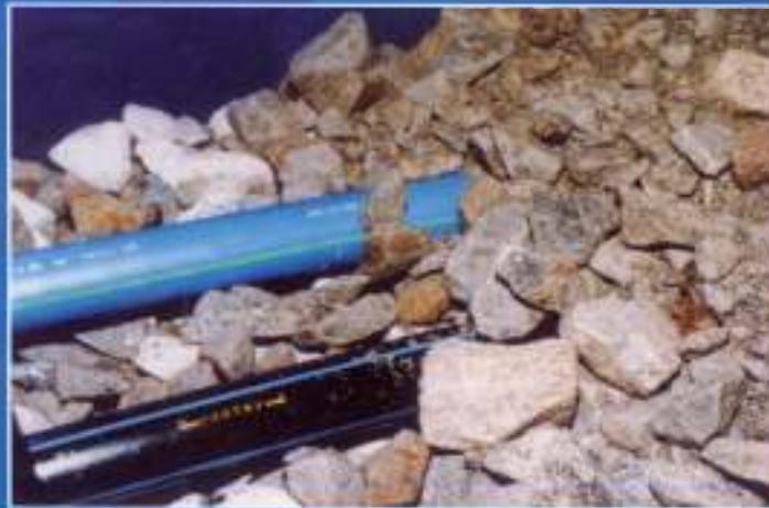
Sand bed free installation possible up to core dimensions of \leq 63 mm
