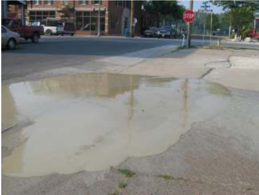
Inadvertent Drilling Fluid Return “Frac-out”
