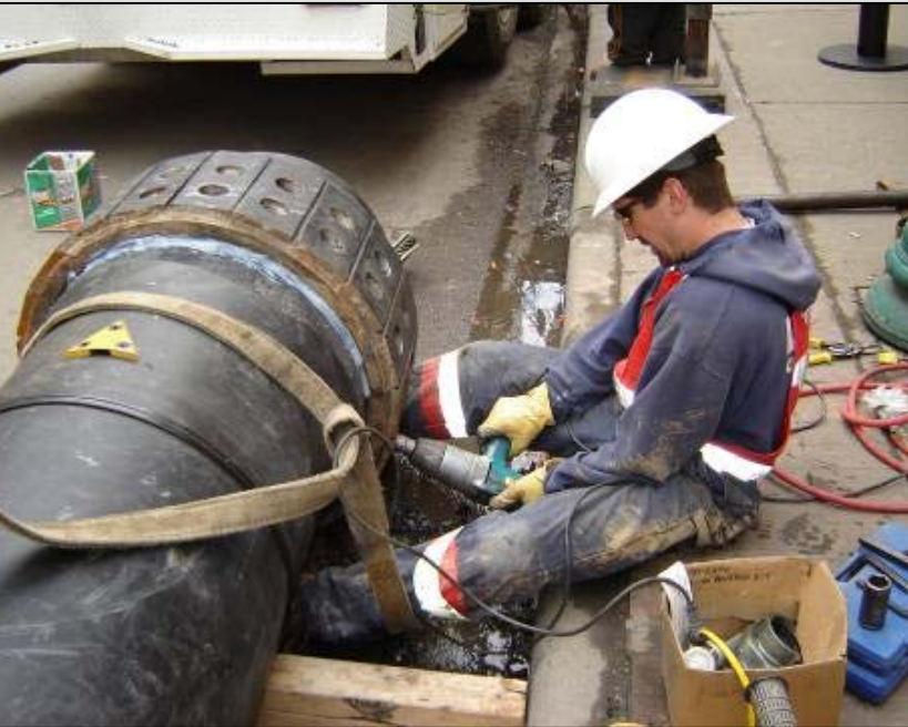
Bolting down burst head onto new HDPE replacement pipe
