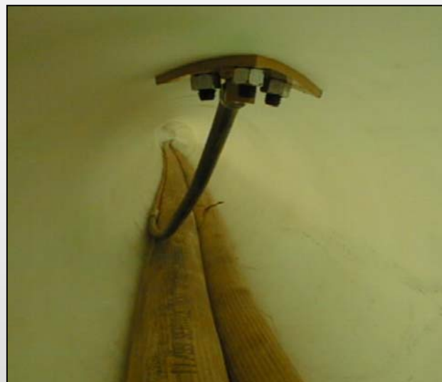
Lubrication feed line inside replacement pipe
