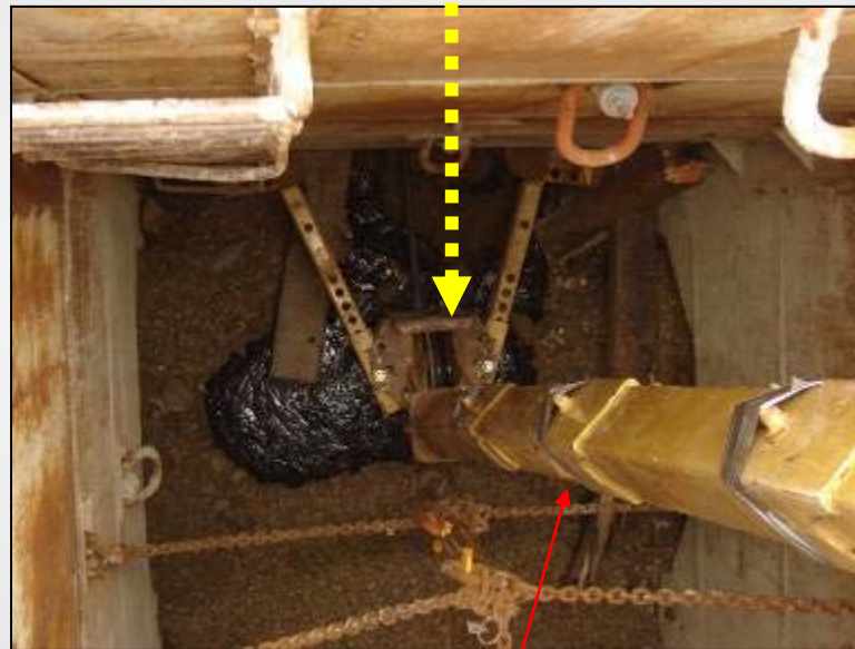
Down leg braced against shoring box
