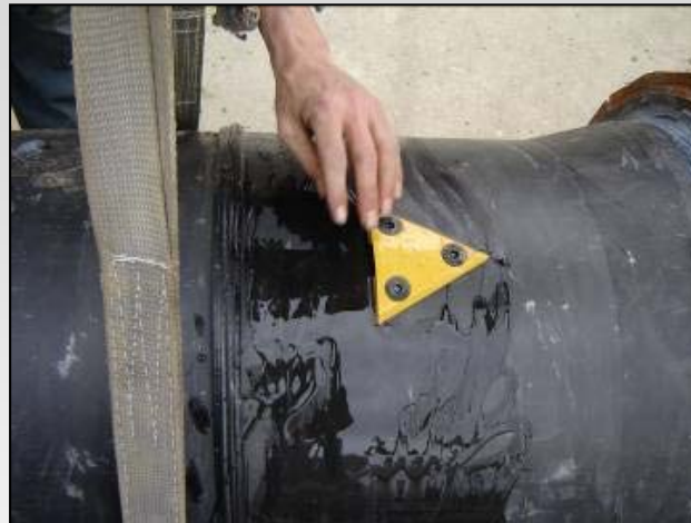
Checking lubricant quality and flow before pipe bursting
