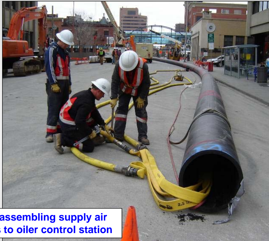
Oiler control station – supplies lubricated compressed air to activate pneumatic hammer
