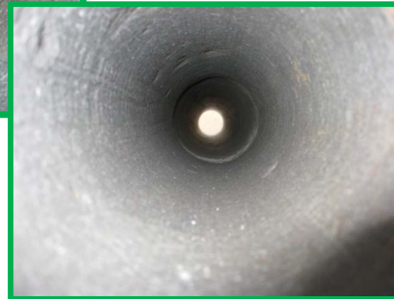
Fully prepared for liner bonding
