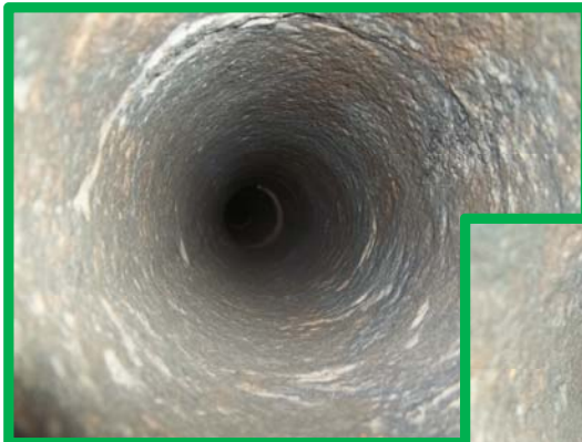
Bitumen liner being removed
