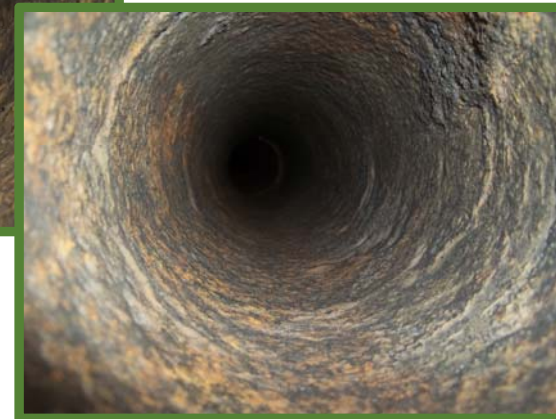
Full tuberculation removal, bitumen liner visible
