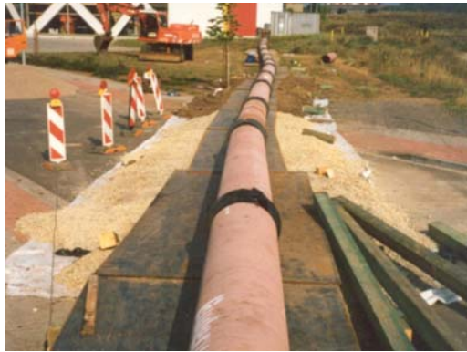
Fig. 11. Pre-assembling onto sheets of metal
