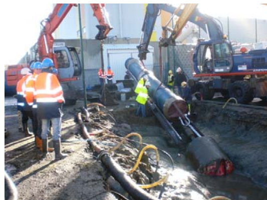
Fig. 18. Grobbendonk – Installation ramp
