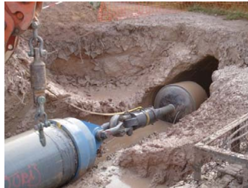
Fig. 14. Alzira – Starting pulling process
