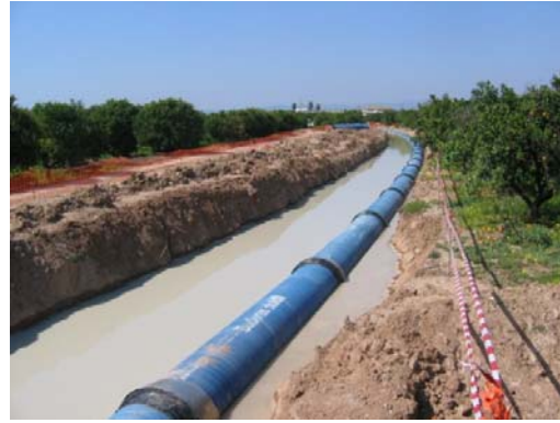
Fig. 12. Pre-assembled with flooded pipe trench
