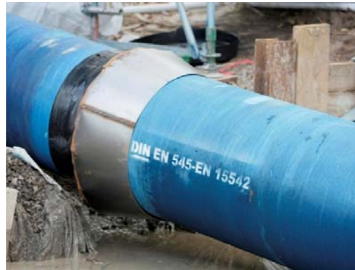
Fig. 5. Socket protection with sheet-metal cone
