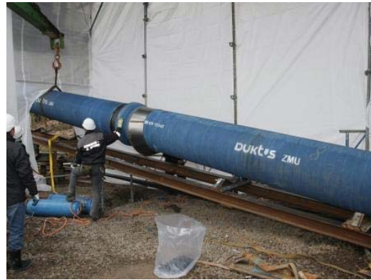
Fig. 16. Installation via ramp
