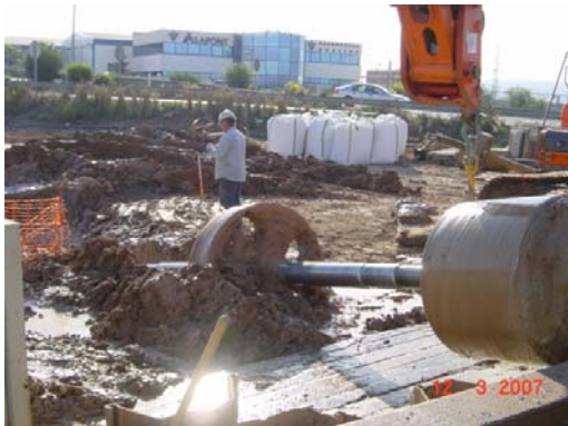
Fig. 13. Alzira – Widening borehole
