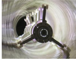
Figure 7. Liner Being Cured with U.V Lights
