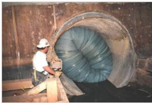
Figure 6. Liner Being Installed
