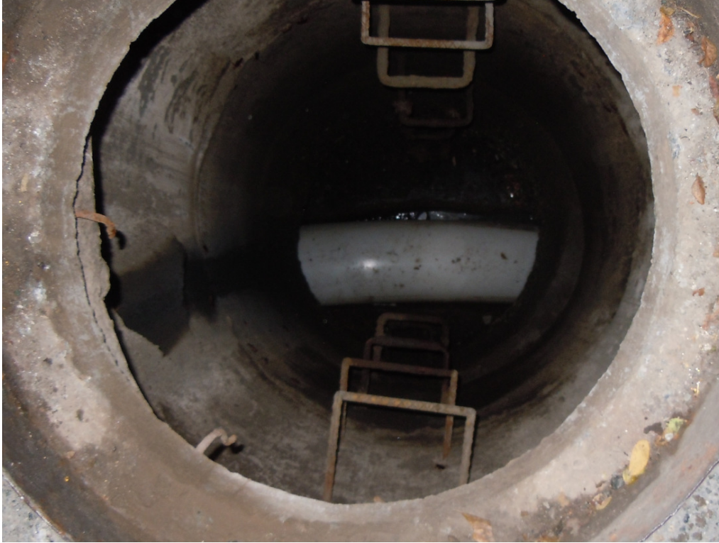
View in an intermediate manhole after reversion.
