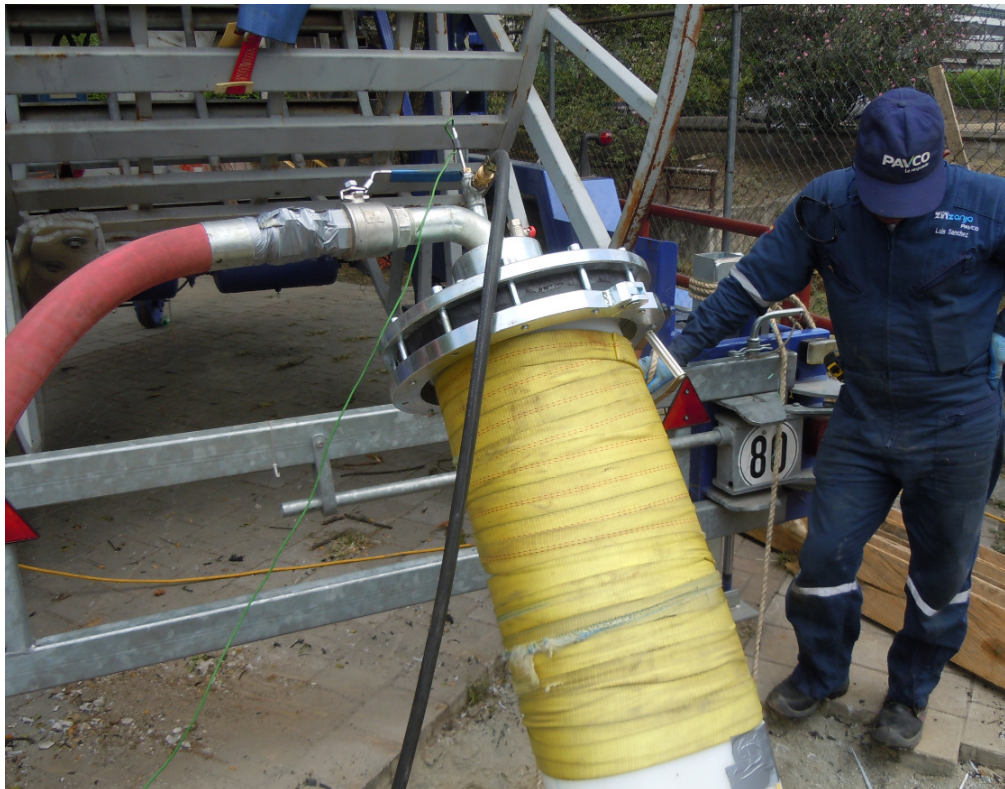
Reverting the pipe by using steam. The parameters, pressures and temperatures are monitored during the reverion process. (This is a non-curing process. It just wakes up the materials memory)
