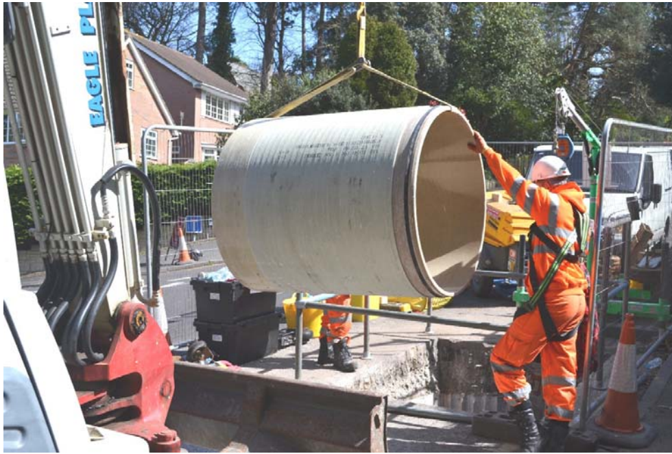
Figure 9. Amiantit SRM TYPE1 GRP linings imported from Poland.
