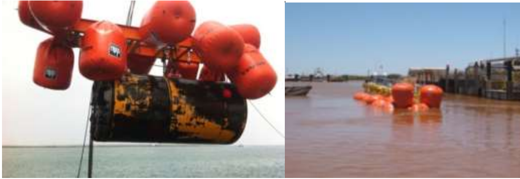
Figure 8 recovery of tunnelling machine via airbags, lifting by crane in harbor
