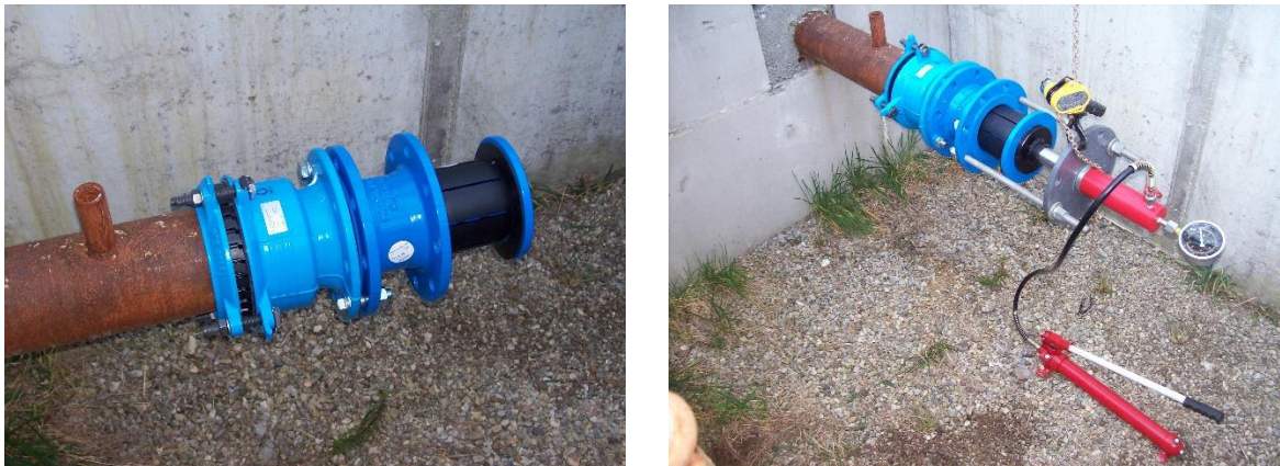
Figure 2: Installation procedure of the low pressure termination fittings
