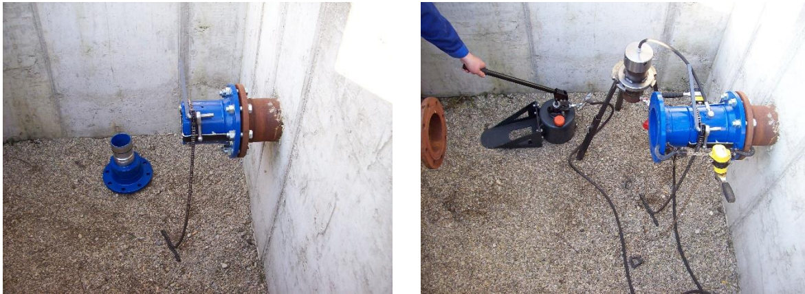
Figure 4: Installation procedure of the medium and high pressure termination fittings
