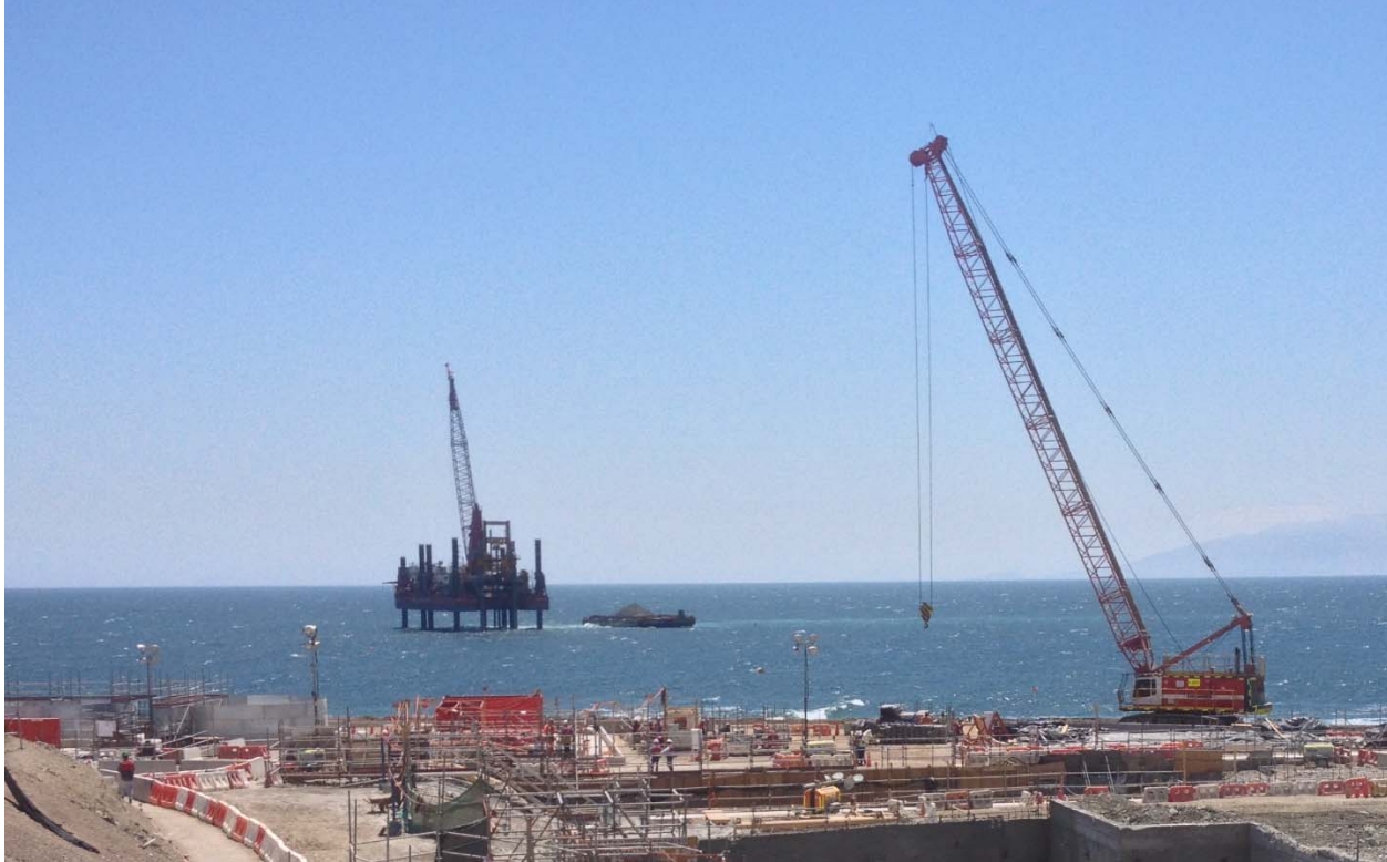
Figure 8. Construction site view
