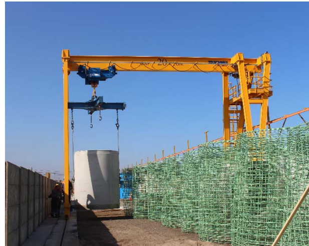
Figure 3. Jacking pipe precast
