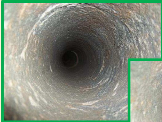
Bitumen liner being removed
