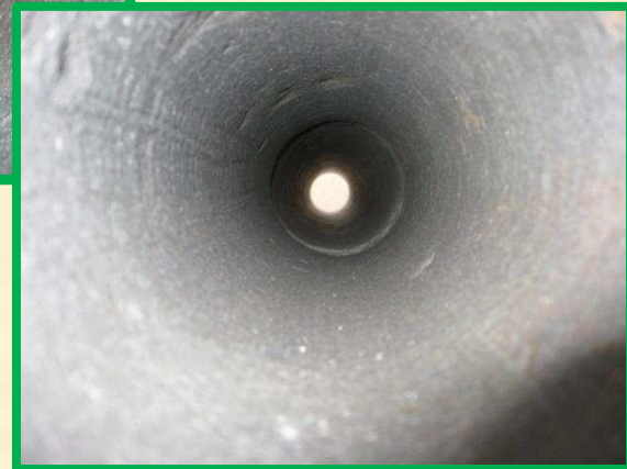
Fully prepared for liner bonding
